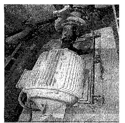
Main fire pump 75HP for fire hydrant
