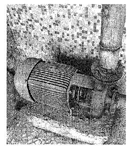
Booster fire pump 7.5HP at Terrace for pressurizing hydrant riser.
